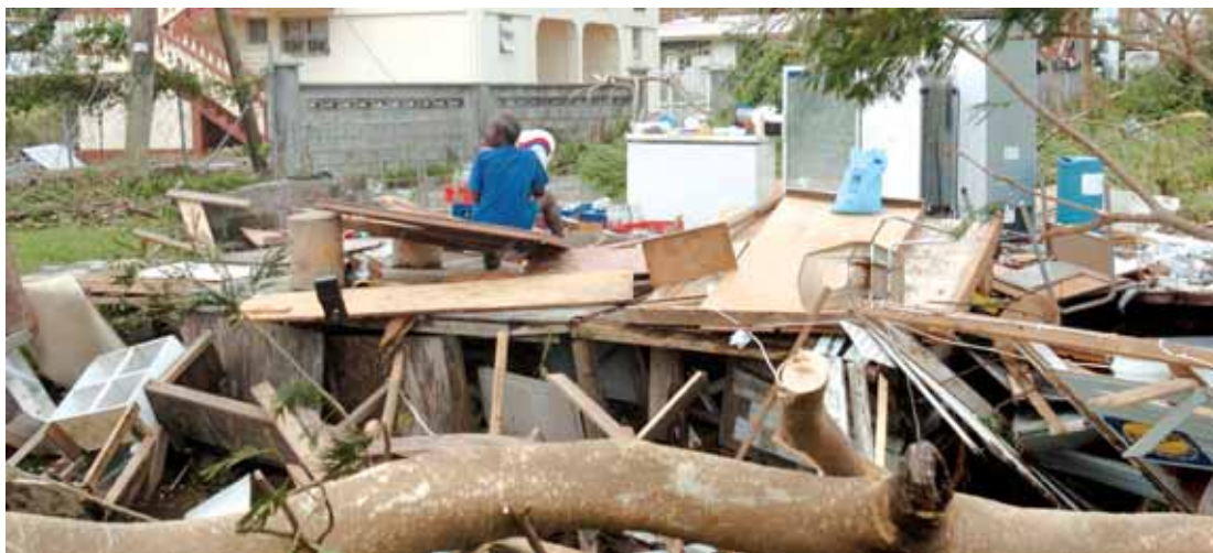
Hurricane Ivan in September 2004 destroyed 90 per cent of Grenada's buildings.
