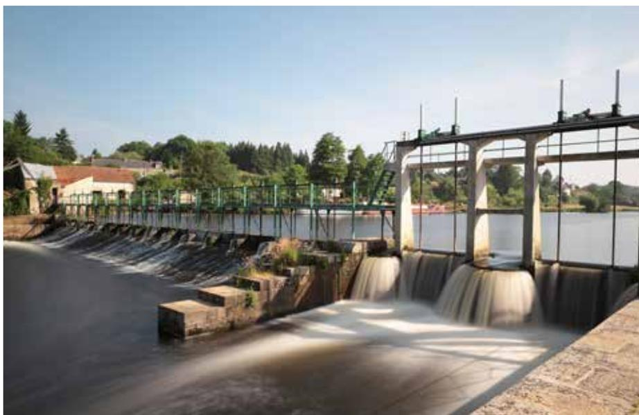
**Figure 14. Water management – spillway for a reservoir**
