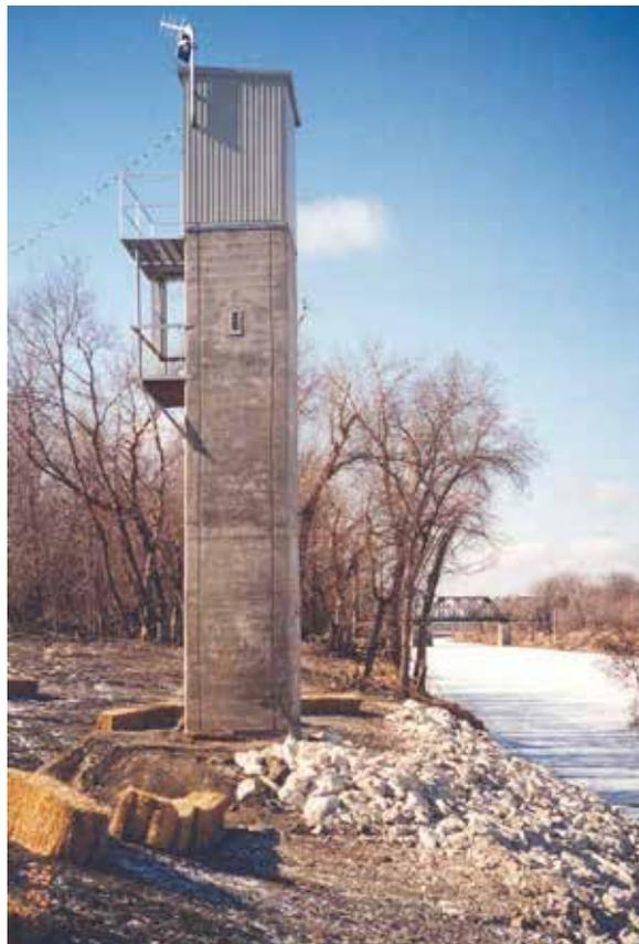
**Figure 6. Hydrometric station built to withstand a large range of water levels**
