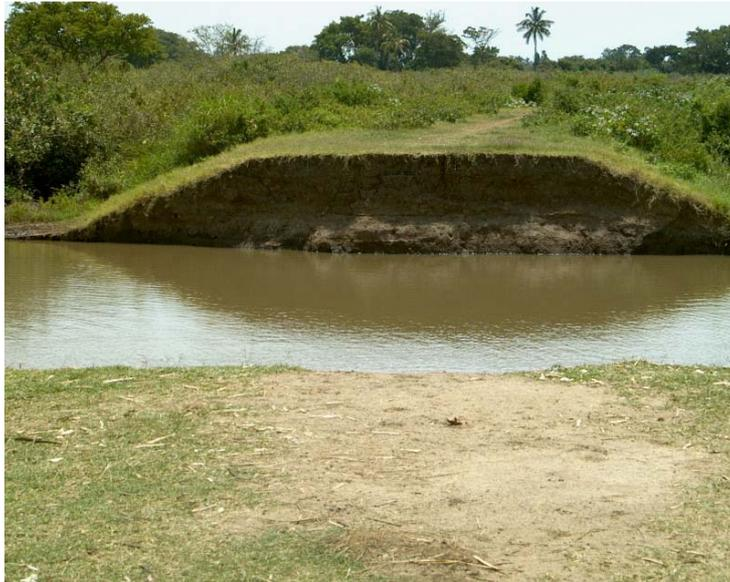
**A broken dyke on the River Nzoia caused by the August 2003 floods in the Budalang'i area.
